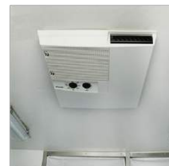
AIR CONDITION UNIT WITH HEAT STRIP
