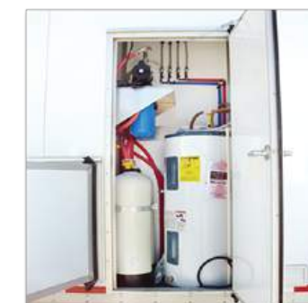
MICRON & LEAD FILTRATION SYSTEM
