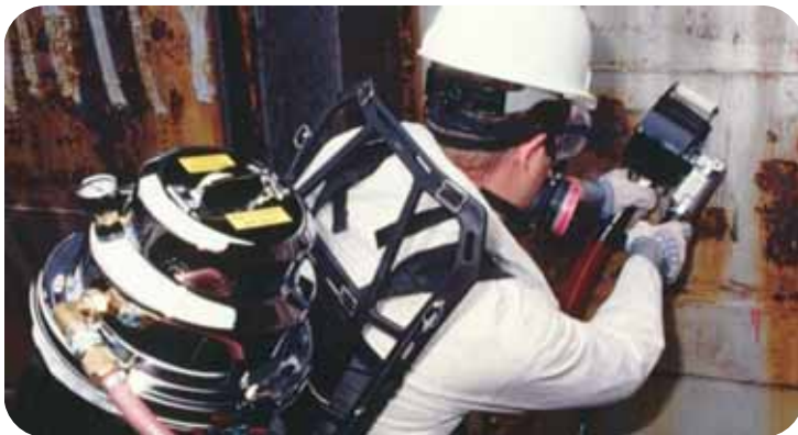
Air Backpack model with RotoPeen tool removing rust from a steel structure.
