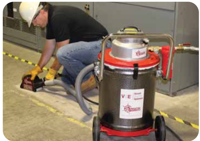
Electric model with Roto Peen tool removing coating on concrete
