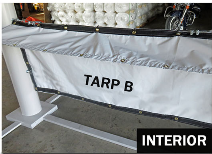
This is a view of Tarp B viewed from inside the work area.
